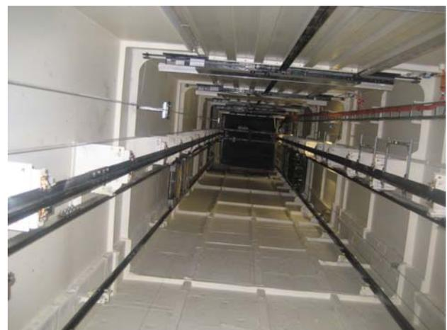
Fig. 2 Pendulum in lift shaft, view looking upwards
